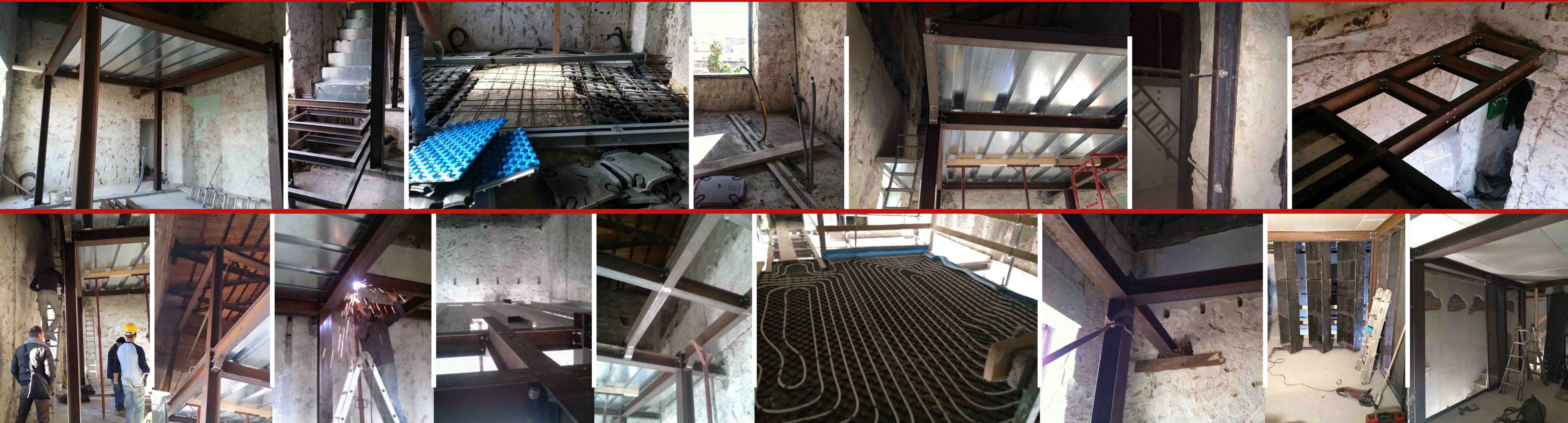
UNDER CONSTRUCTION PICTURES
